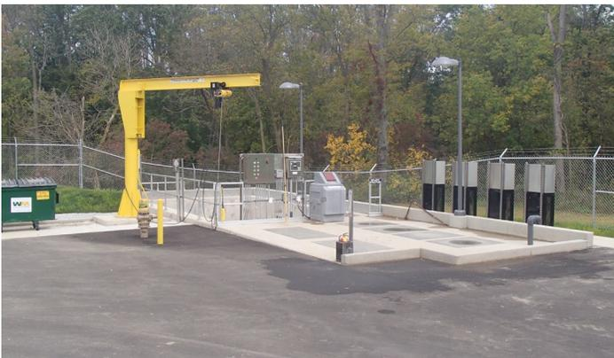
*New headworks structure including fine screening and raw sewage pumping.*
