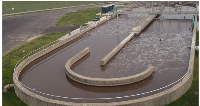
*Modified oxidation ditch with new blowers, fine-bubble diffused air, and submersible mixers.*
